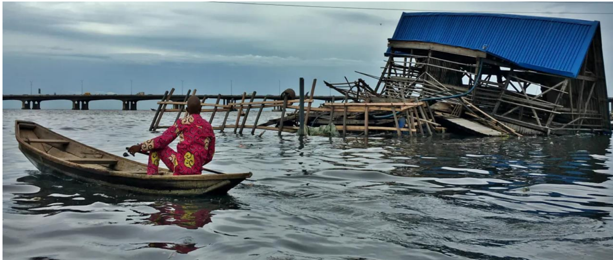
Figure 15: shows a local man looking at the buoyant school construction collapse following a heavy rainfall in Lagos. Photography by Allyn Gaestel. The Atavist Magazine. Accessed online: https://magazine.atavist.com/things-fall-apart-makoko-floating-school/
